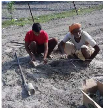
19(b) Step 2: Tying the GI wire to the anchor bricks
