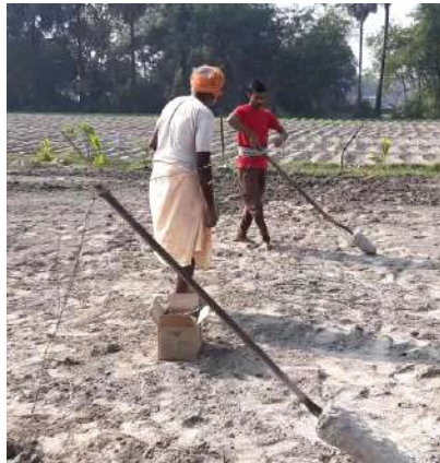
19(e) Step 5: Erecting the slanted end poles
