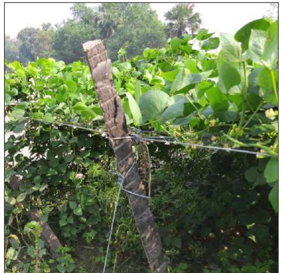
Fig. 18: End pole tied to the ground level support using GI wire
