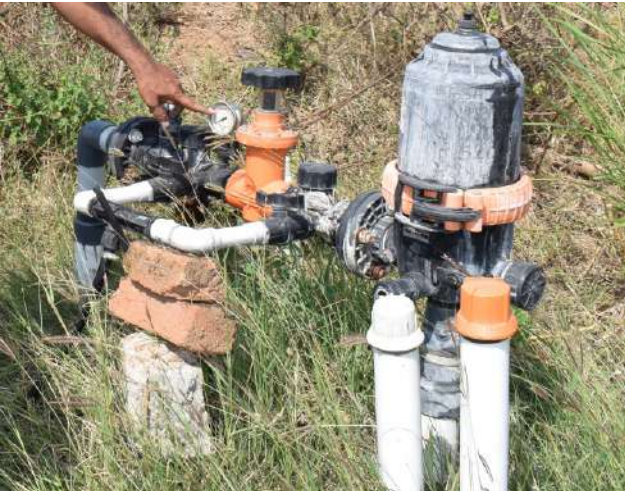
Fig. 39: A drip irrigation unit with a venturi for fertigation
