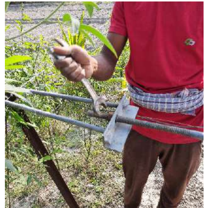
19(f) Step 6: Tightening the GI using a turnbuckle
