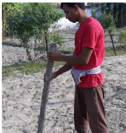
19(h) Step 8: Erecting internal bamboo poles
